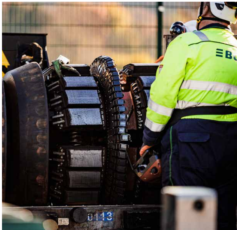
Smart inspection robot for inspecting the TAG pipeline system.
