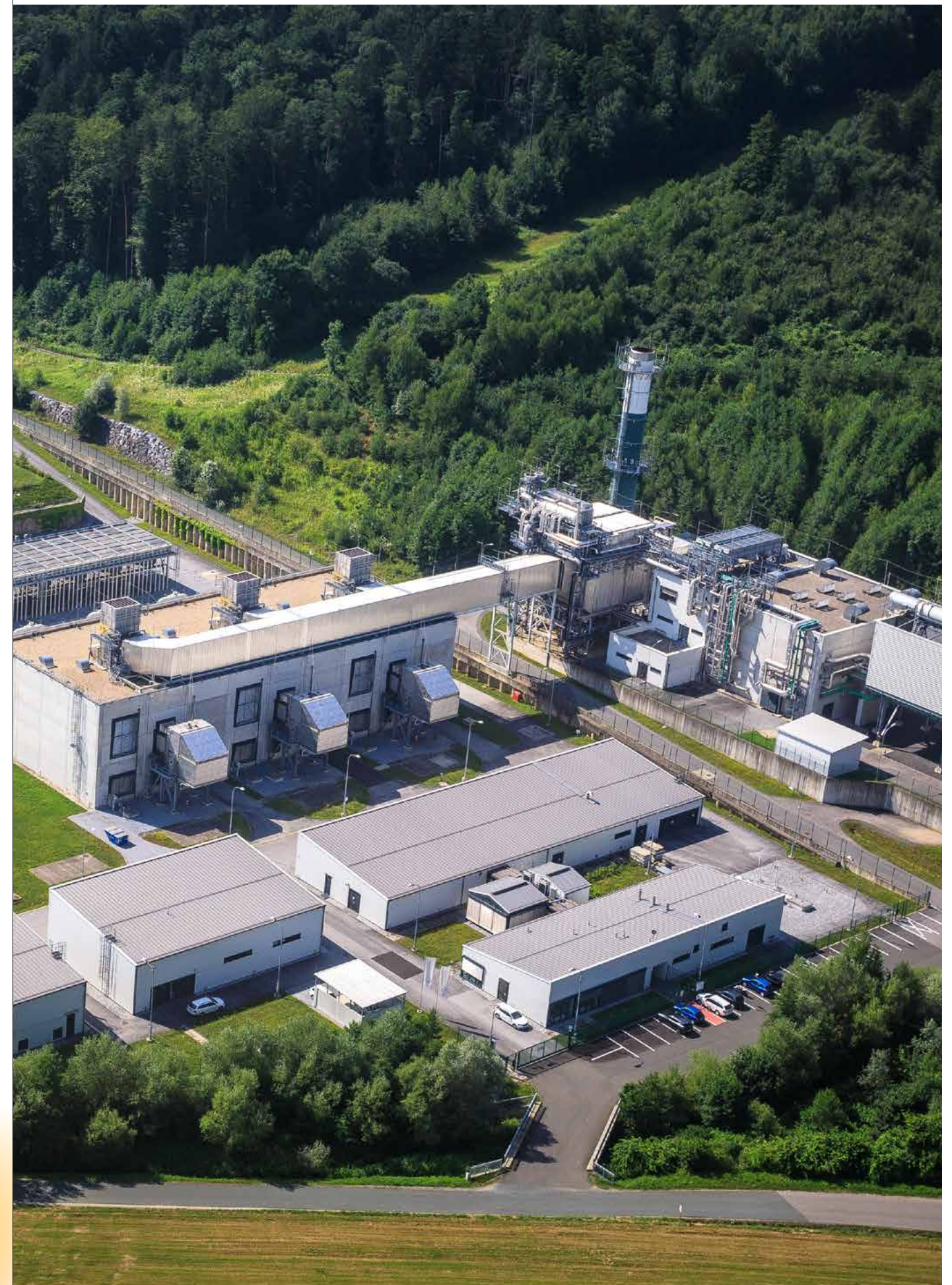
Compressor station and waste heat recovery unit in Weitendorf.
